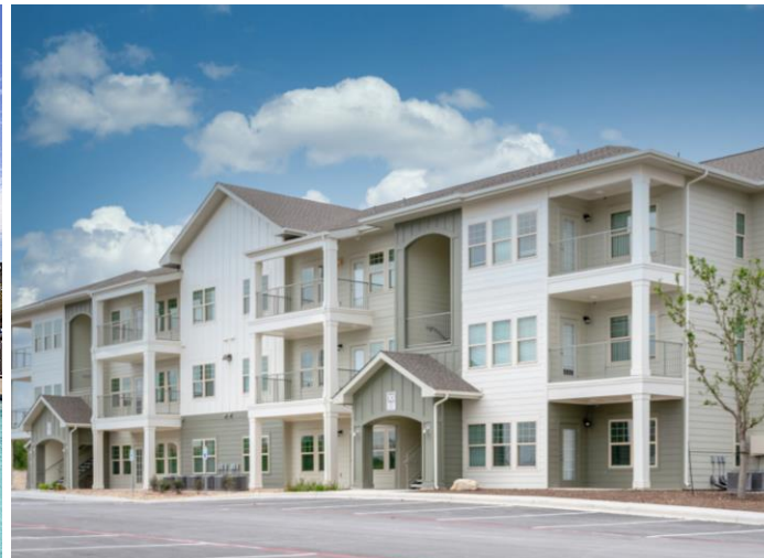
EXETER PLACE 248 UNITS BUILT 2020
